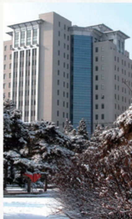
The exterior of the Library
